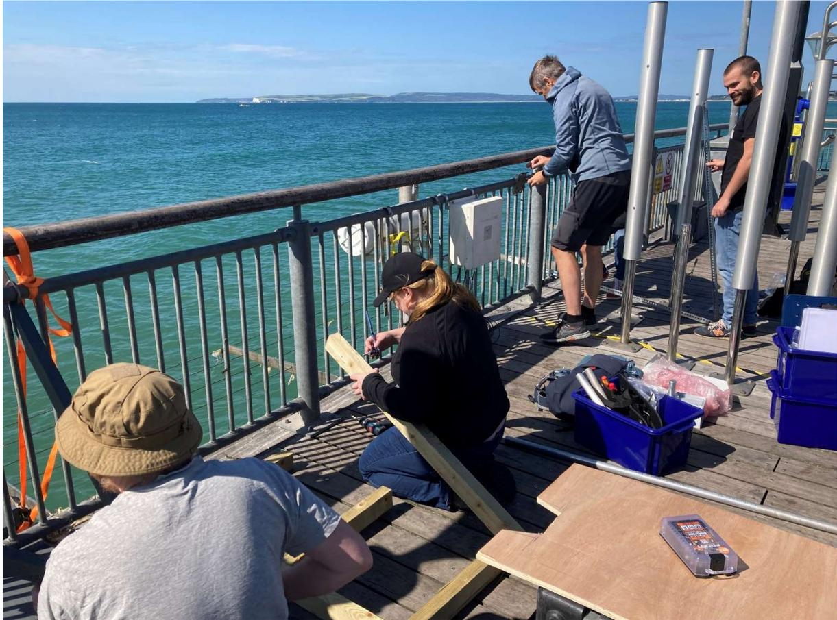
Figure 3 Radiometers being installed for measurement of the sea at the tip of the pier
