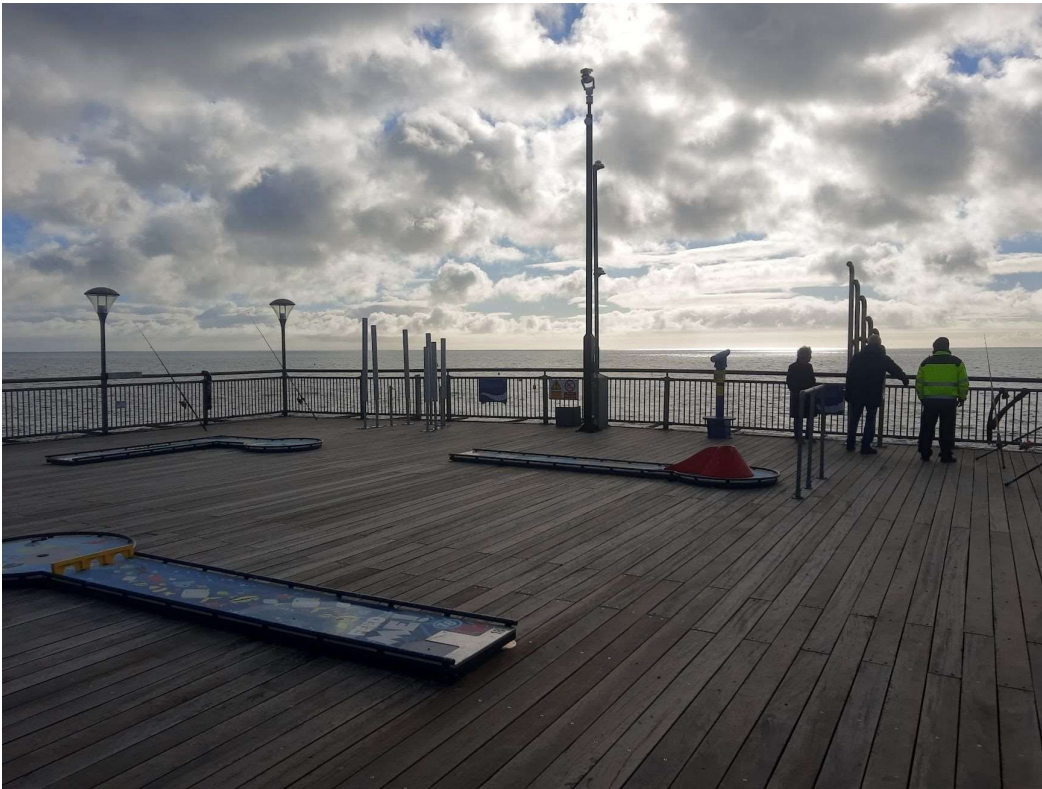
Figure 4: Boscombe Pier, pier head.
