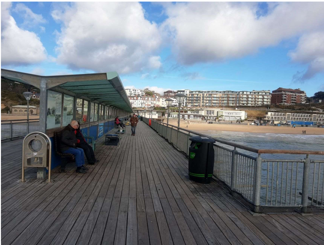
Figure 3: Boscombe Pier, looking back from the pier head.
